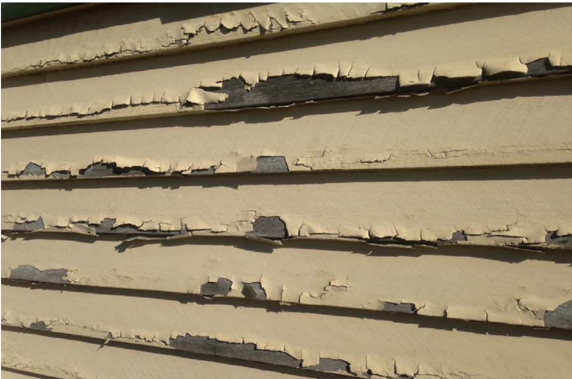
Photograph 4 – Example of peeling external paint.
