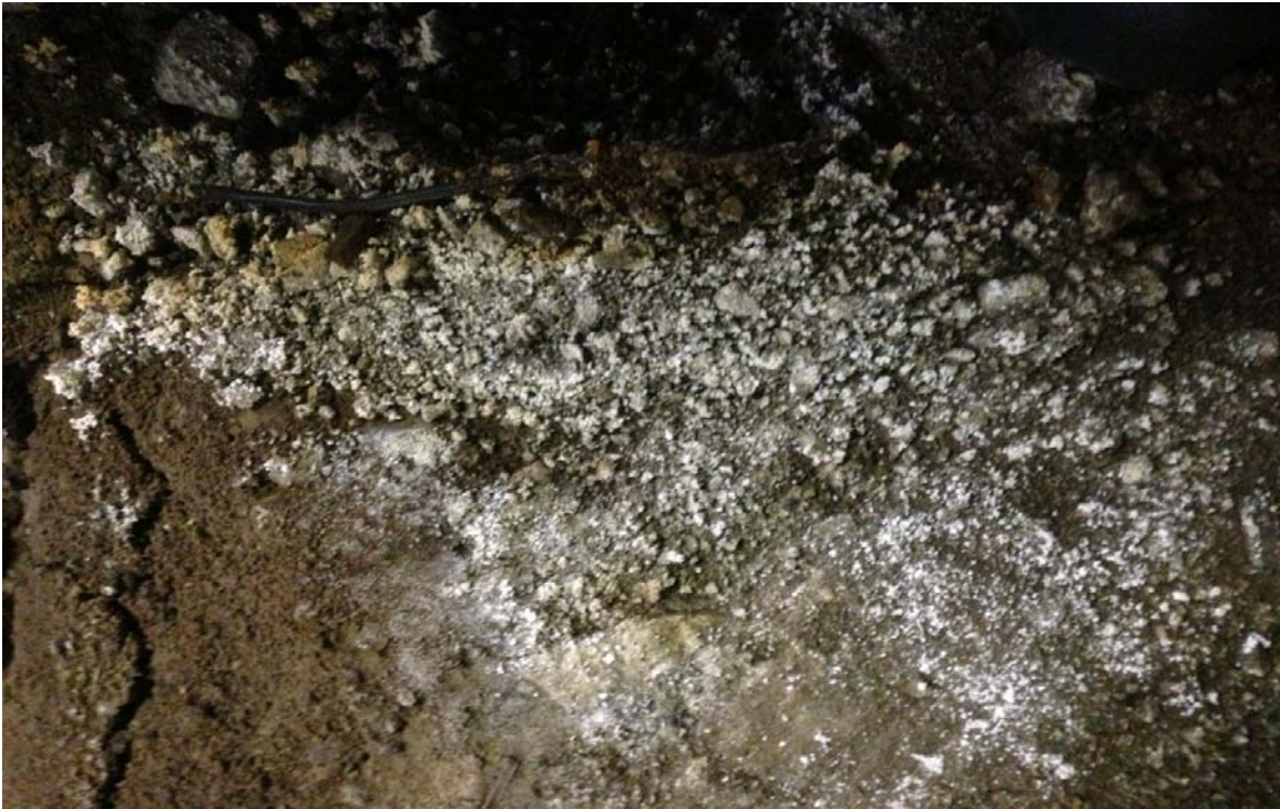
Photograph 3 – Salt crusting beneath southern building.
